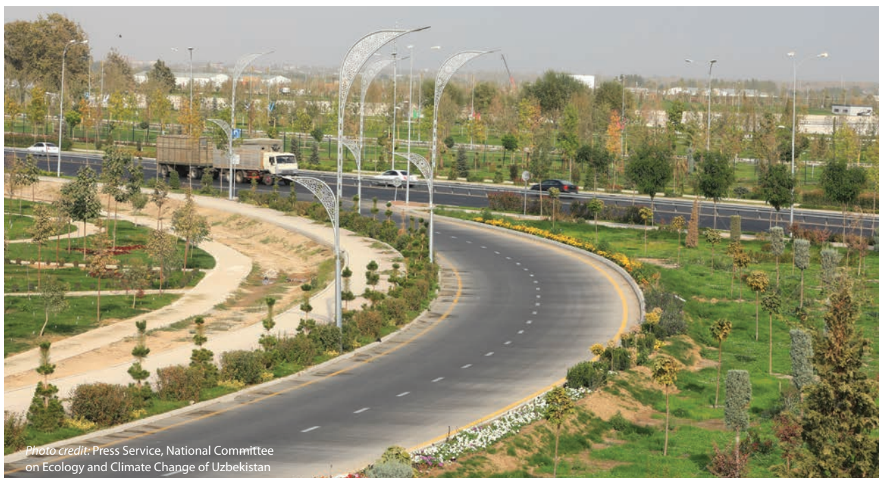
Photo 2.1: Green Belt within the infrastructure of Uzbekistan's modern highways
