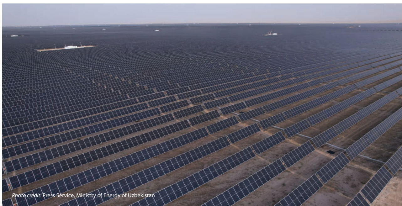
Photo 2.2: Solar Park in Kamashin District, Kashkadarya Region, Uzbekistan
