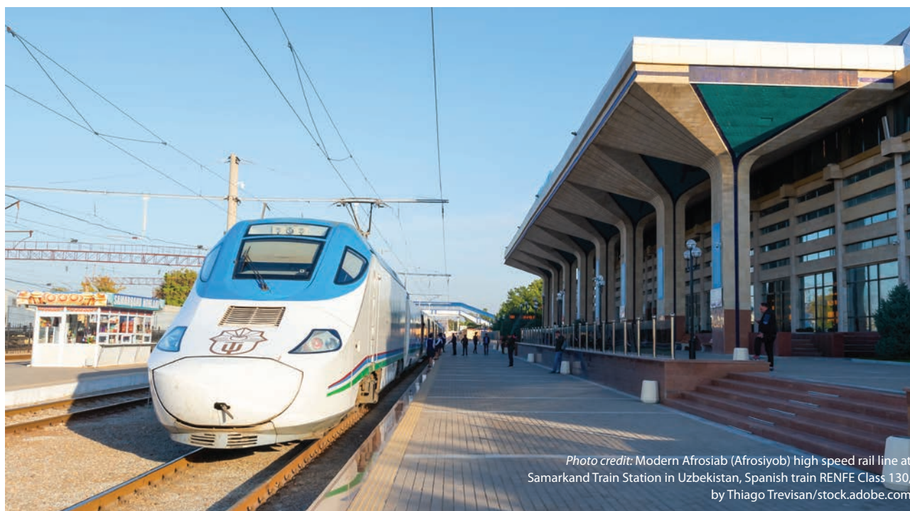
Photo 3.4: High speed train, Samarkand Train Station
