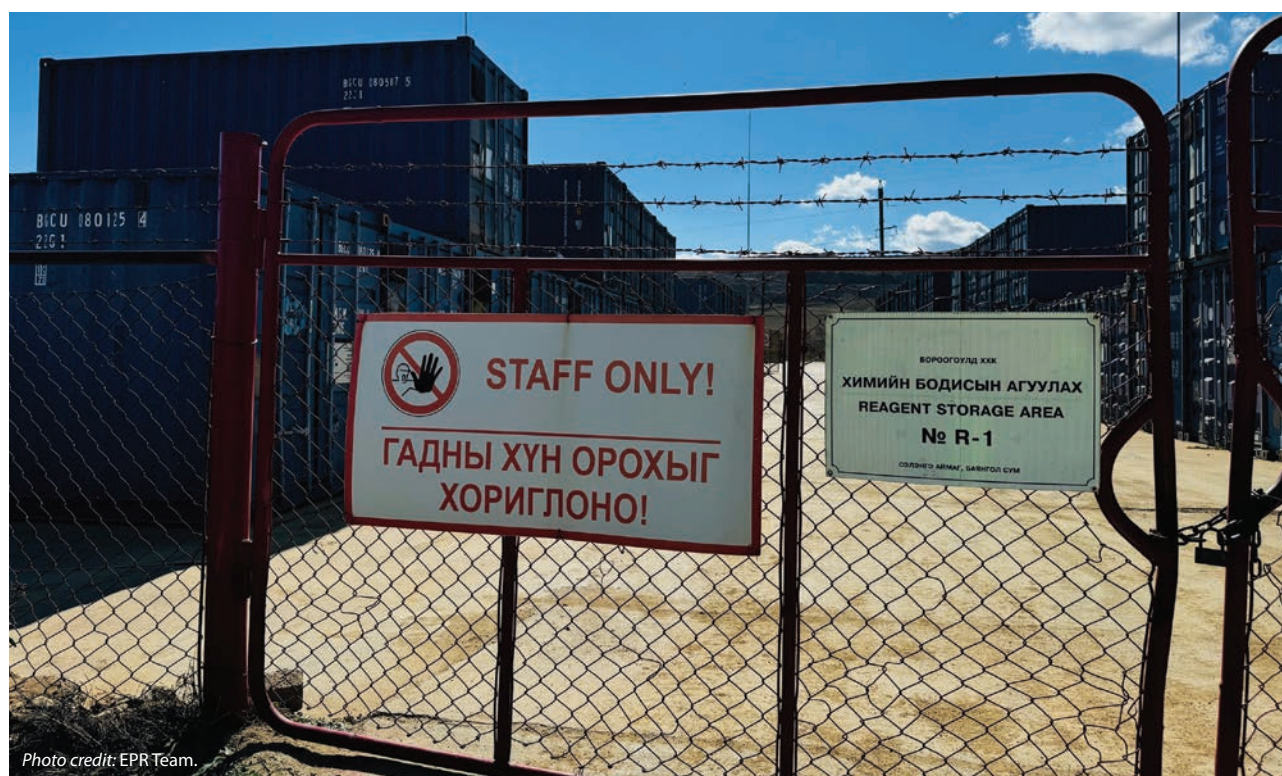
Photo 16.2: Chemicals storage pad, Boroo gold mine
