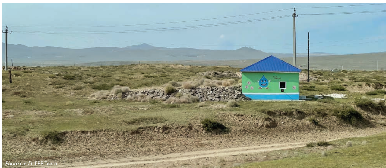
Photo 6.2: Water utility building in the countryside
