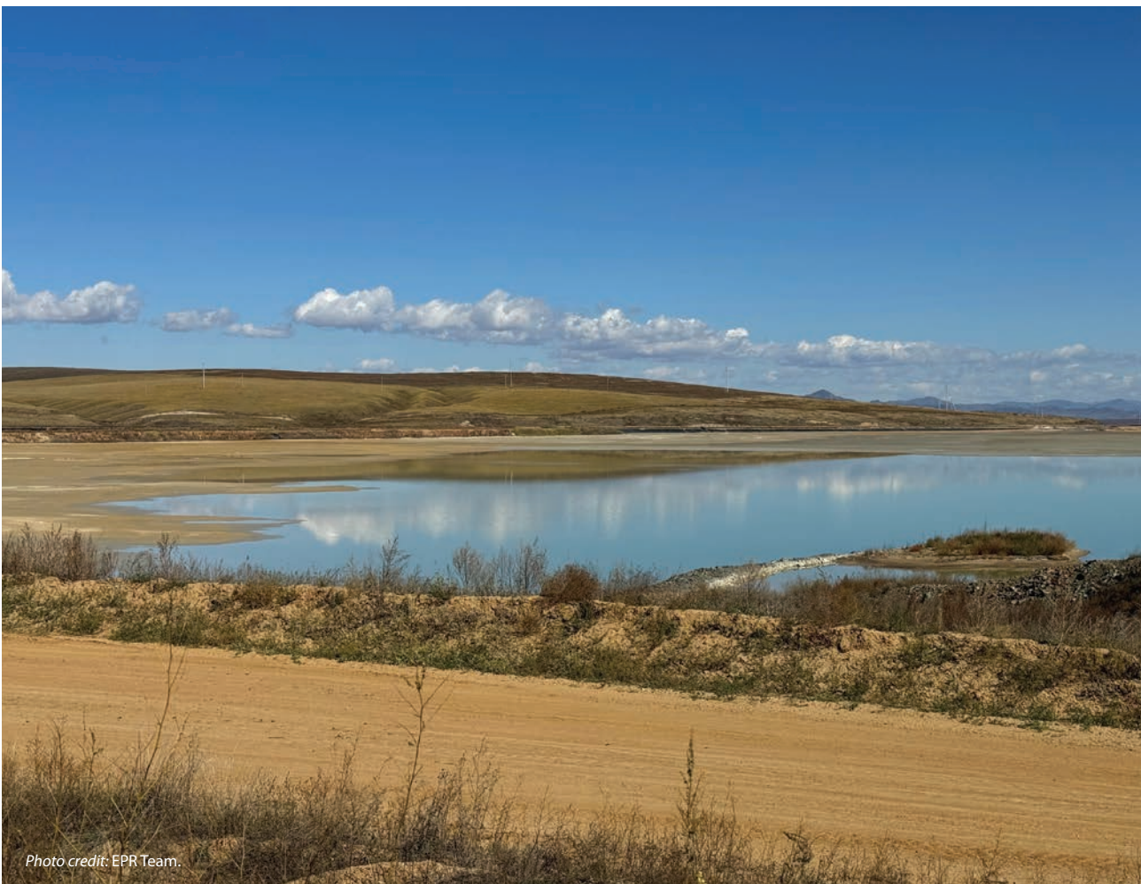
Photo 16.1: Tailings dam, Boroo gold mine
